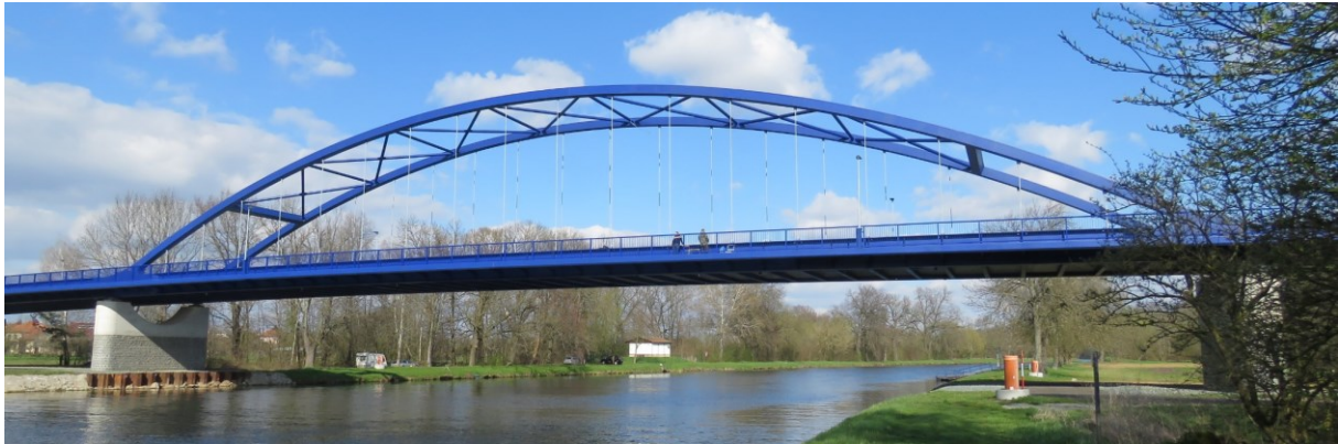
Figure 1. The view on the third span of the bridge where the structure is reinforced by the arch.
